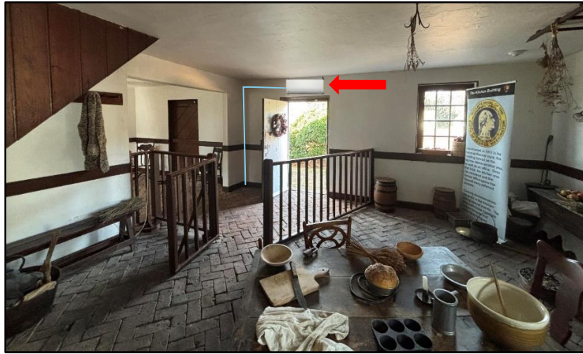
Figure 1. Photo simulation of proposed indoor wall-mount unit #1 in demonstration space. Blue line shows trajectory of line set. Photo is to scale.
