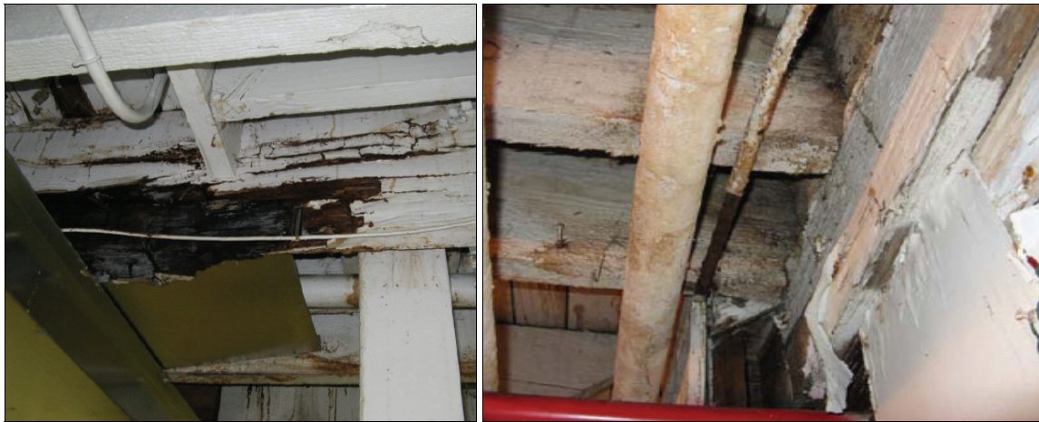
Figure 1-3 Examples of deteriorated floor beam and wood decay at structural members of the north wall and ceiling, basement level.
