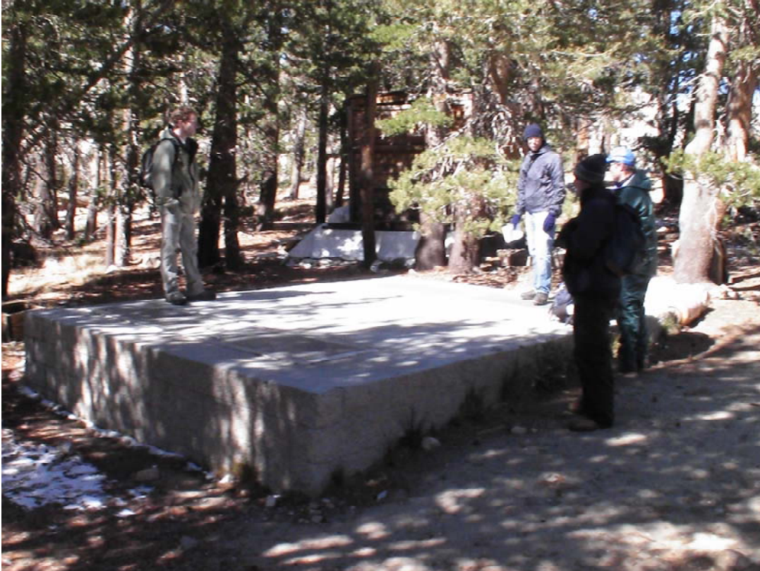
Photo#2: 6,900 gallon concrete & masonry block septic tank.
