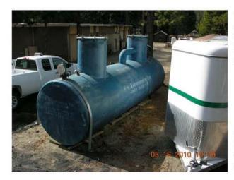
This photo is the two chamber separator that will be installed. The tank is double walled with an interstitial space monitoring port for installing leak detection sensors.
