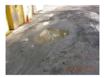
Photo above is the top of existing wash rack showing standing water at the inlet. The access hatch to the existing failed oil separator can be seen just outside of the wet area. The manhole connection to the sanitary sewer system is at the top of the photo.
