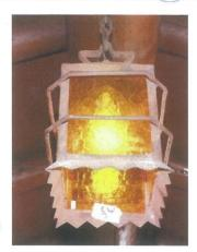
**Condition:** Wire is concealed beyond porcelain socket but exposed wire above loop is old and brittle. Fixture is not internally grounded. Socket is loose. Tabs are broken. Overall structural integrity of lantern is sound. Original brown paint is worn.
