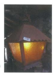
**Condition:** Wire is concealed beyond porcelain socket but exposed wire above loop is worn and brittle to the touch. Fixture is not internally grounded or polarized. Socket is loose. Overall structural integrity of wall sconce is sound. Original brown paint is worn.
